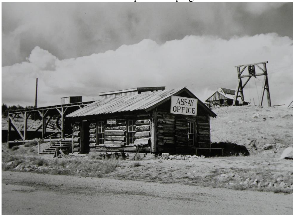
H4. Office in place. Original Mining Mill visible to left. Head House and Gallows Frame visible to the rear. c.1959 (Compare to current photo #21).
