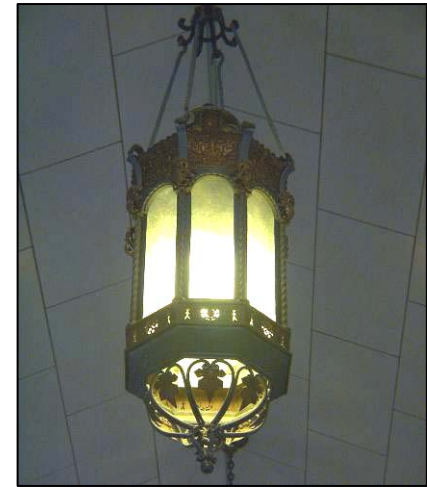
Original fixtures should be retained when updating electrical systems.
