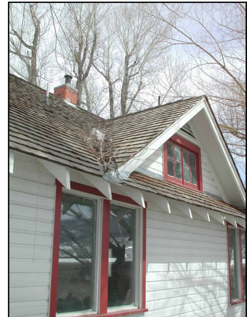
Dirt and debris should be removed promptly from all roof drainage systems.
