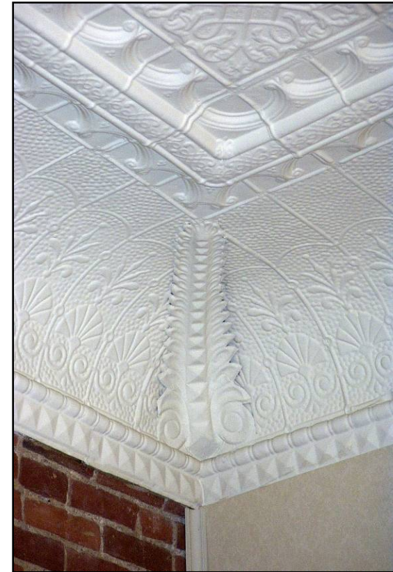
Tin ceilings should be checked for corrosion, staining, and other damage.
