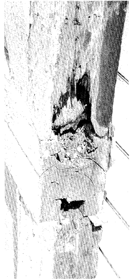
Figure 5. Some internal core deterioration was masked by sound surface wood. Water entering the connection of the post and beam framing rotted out the mortise and tenon pockets. These areas were consolidated and filled with epoxy. Photo: Baird Smith, AIA
