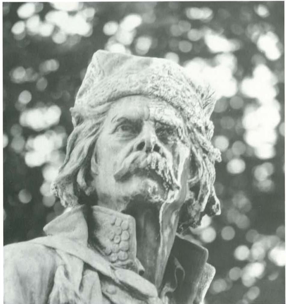
Figure 3. Detail of the west sculpture group, depicting a pair of soldiers. Left half of the face has been blasted and presents a more even appearance than the right half, which has not been blasted and exhibits the light/dark streaking common to corroded statuary. Photo: Dennis R. Montagna
