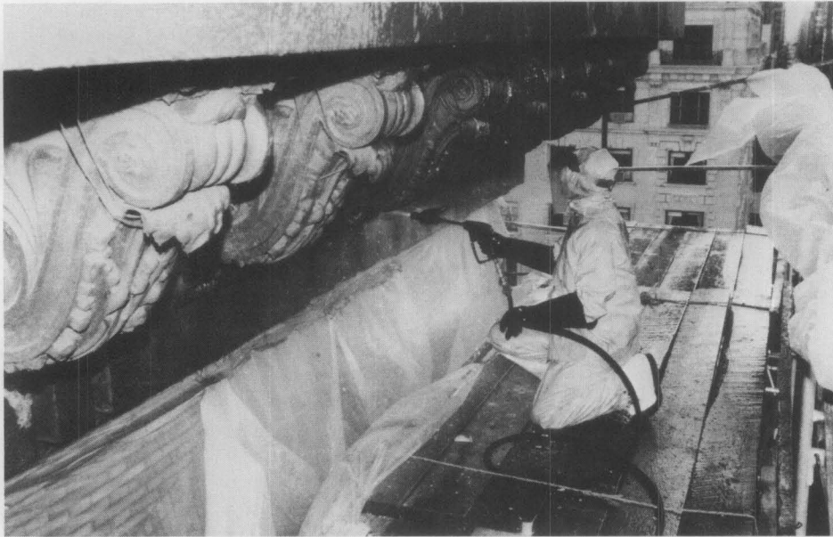
Figure 7. A water spray was used to remove most of the paint from the components of the cornice that were being retained. With the more delicate egg and dart molding, care was required to avoid possible dimpling of the metal. Steps were taken to keep water from collecting inside the cornice. Photo: Michael Devonshire.
