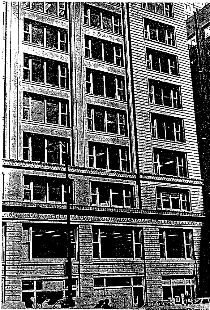
Figure 1. The Marquette Building has both Chicago-style windows, as shown above on the second floor, and a modified Chicago-style window consisting of two fixed lights in the center section. Photo: Charles E. Fisher
