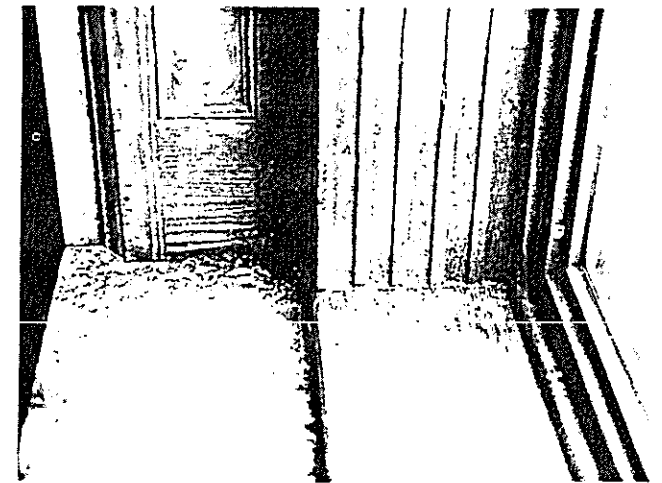
Figure 8. The decorative jamb panel on the left and the interior shutter tracks were unaffected by the installation of the interior storm window shown on the right. Photo: Charles E. Fisher
