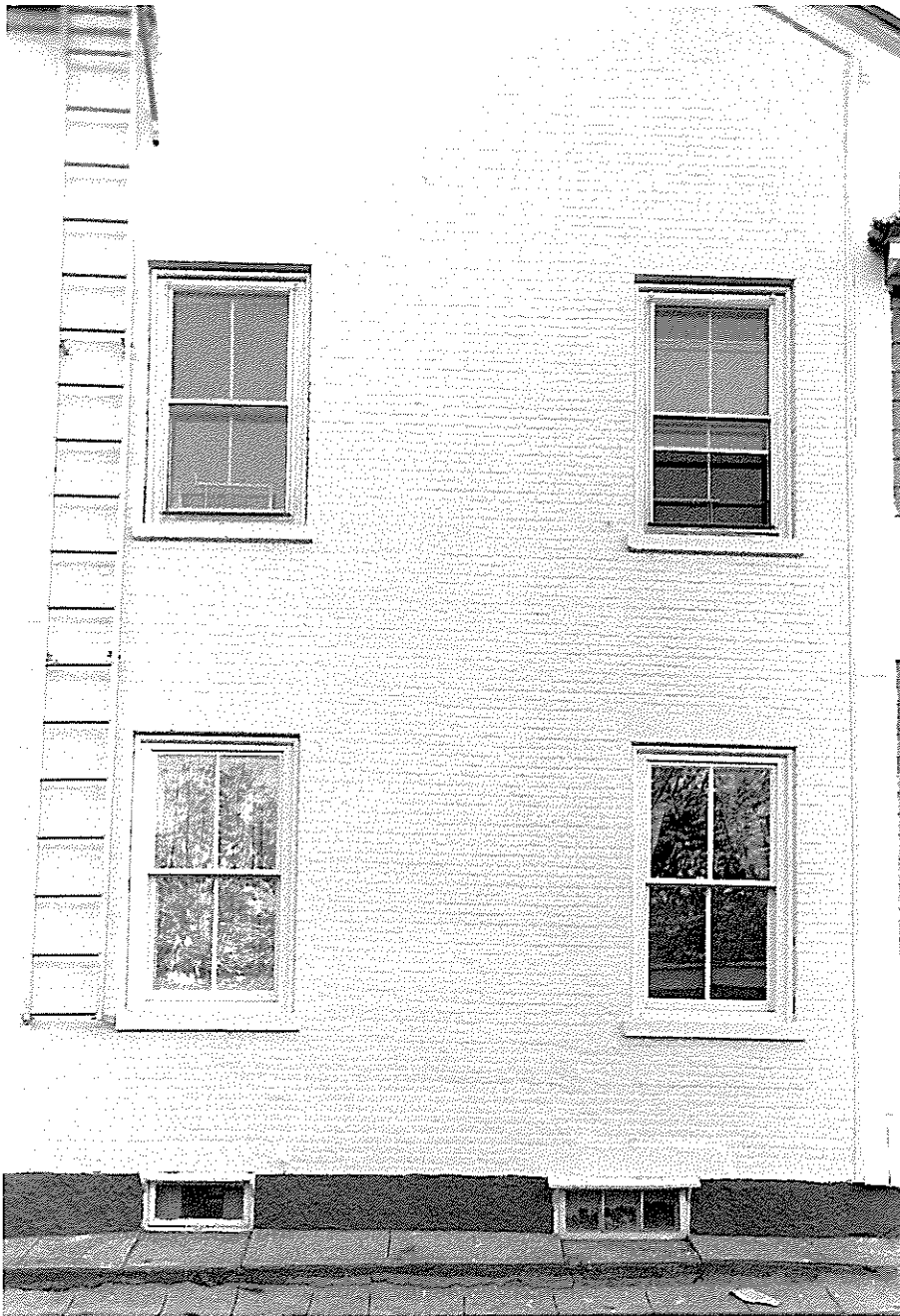
Figure 4. The new wooden windows on the first floor with insulating glass installed closely matched the historic windows which were preserved on the upper floor. Photo: Charles Parrott
