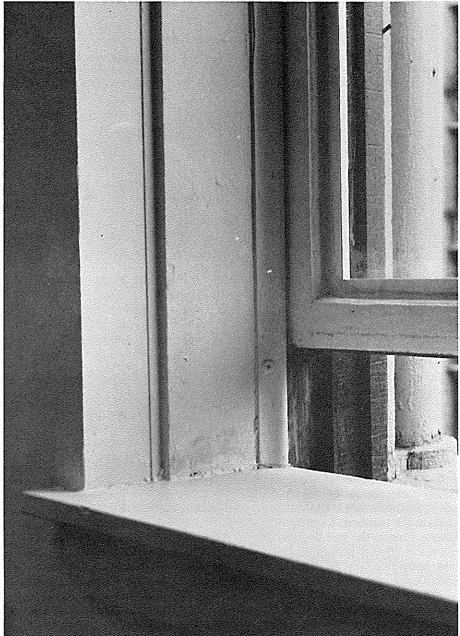
Figure 1. Since the metal spacer placed between the glass sheets is set slightly off the edges of the rails and stiles, the retrofitted insulating unit reduces the historic glass exposure by about 1/2" along all sides. This change on large windows is hardly noticeable particularly once the flat trim piece is glued in place. Photo: Charles E. Fisher.
