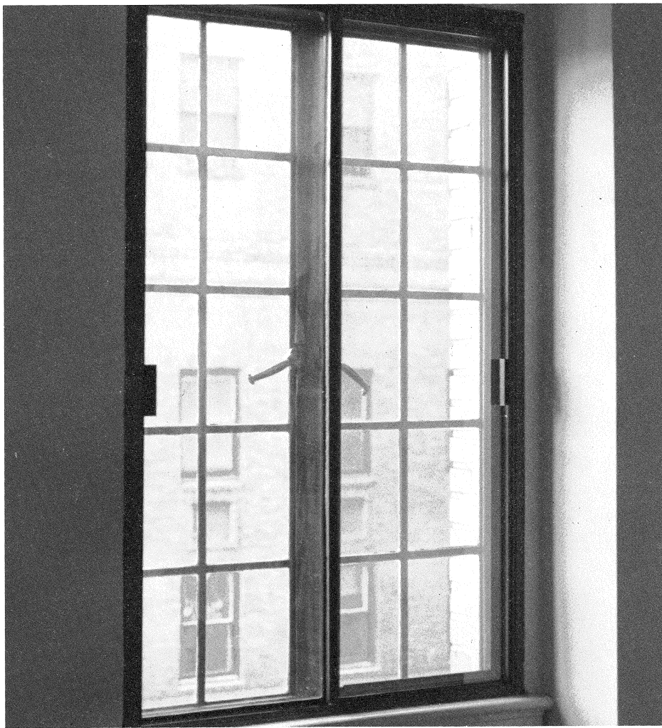
Figure 2. A horizontally sliding storm window unit was installed on the inside of the casement windows for improved energy performance. Photo: Christina Henry.
