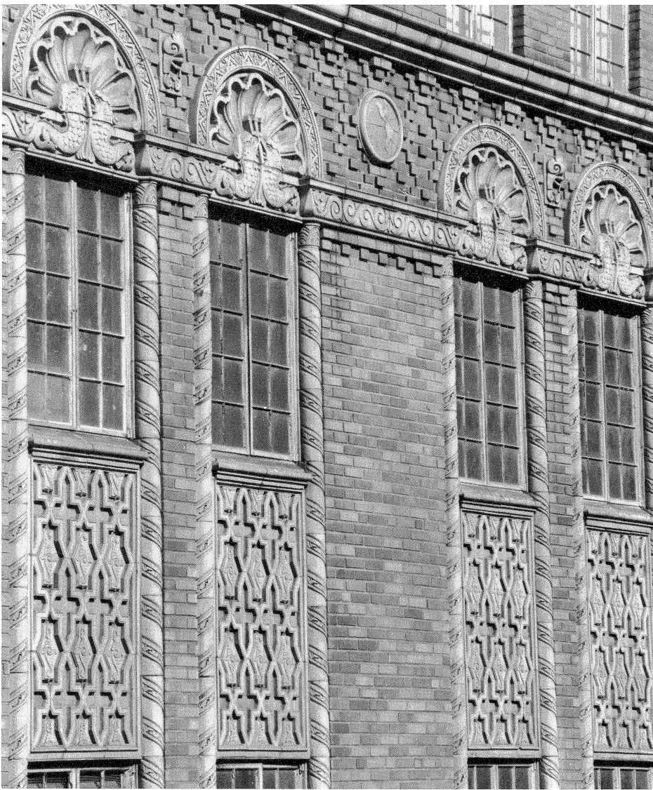
Figure 1. The steel casement windows on the lower and uppermost floors were richly adorned with terra cotta detail. Photo: Mort Bond/National Register Collection.
