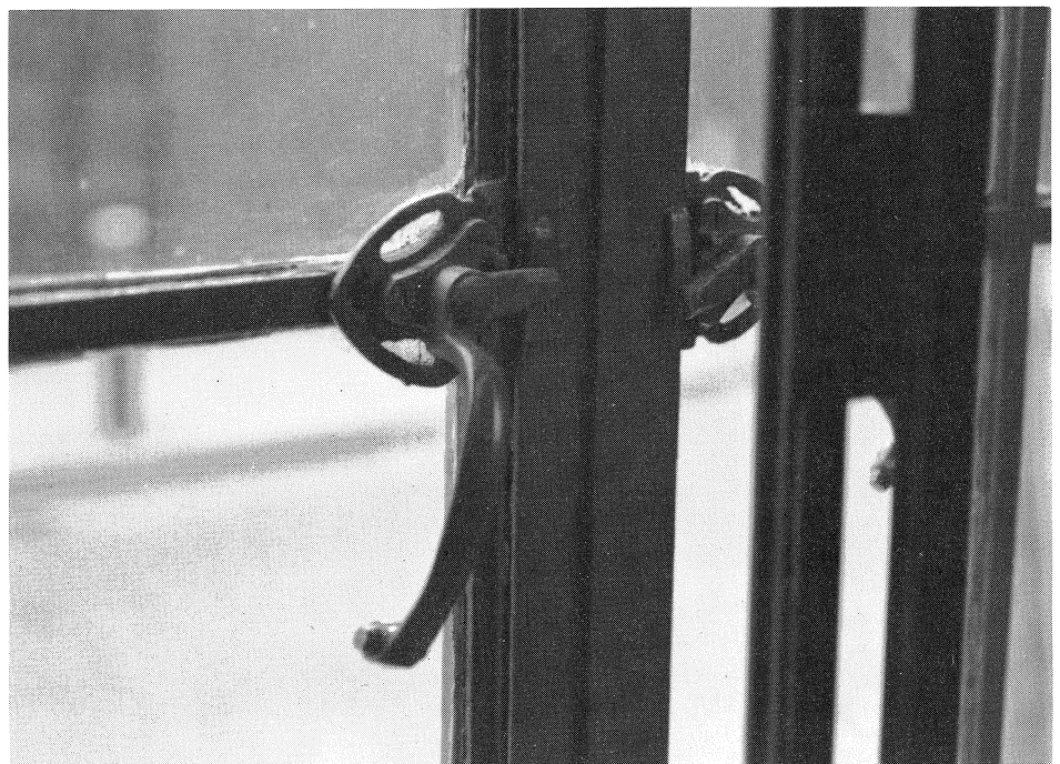
Figure 4. The hardware was cleaned and oiled as part of the maintenance and repair work undertaken on the steel casements. Photo: Charles Fisher.
