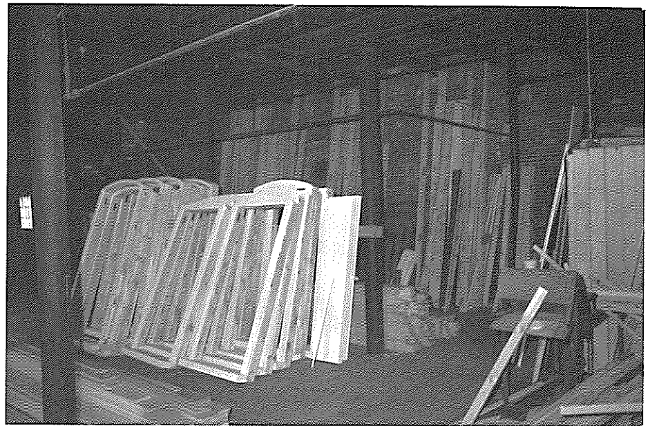
Figure 6. Newly milled replacement window frames awaiting installation. Photo: Christopher Closs
