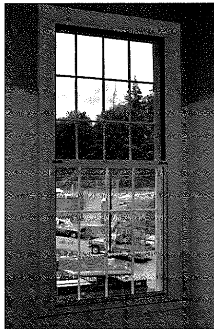
Figure 8. Typical interior aluminum combination storm window unit with insect screen shown at top. Beveled stops around the perimeter were added and the windows were caulked to provide for a good energy seal. Photo: Christopher Closs
