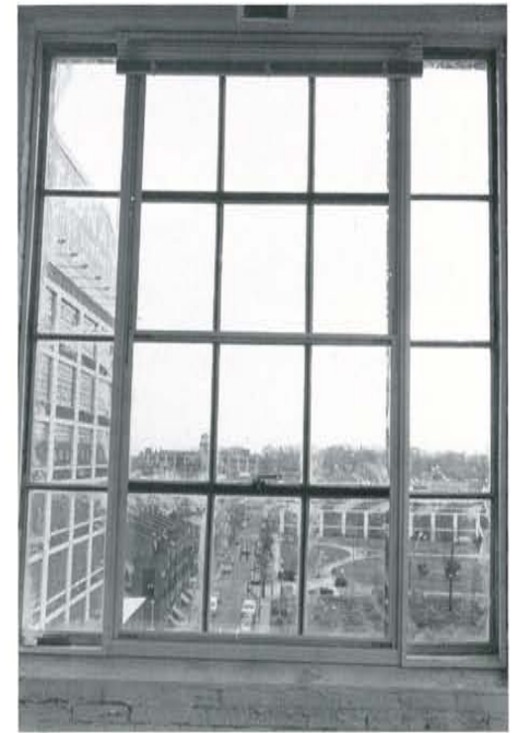
Figure 12. Installed interior triple-track storm window with fixed sidelights. Photo: Clio Group.
