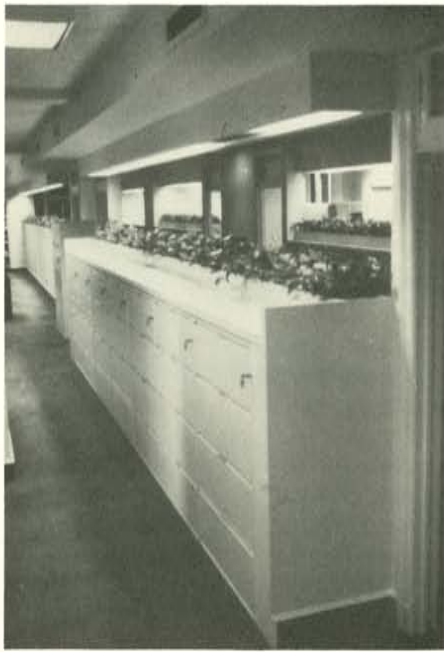
Figure 5. Banks of file cabinets and shelving were set flush against the existing wall and enclosed on the sides and tops. Photo: Nelson & Associates.
