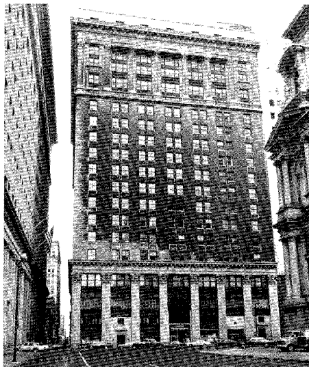
Figure 1. In 1989, just prior to the onset of the rehabilitation project, the Widener Building was showing the effects of 75 years of exposure to an urban environment. Note the lighter color of the left side of the building regularly washed by rain. Photo: John Milner Associates.
