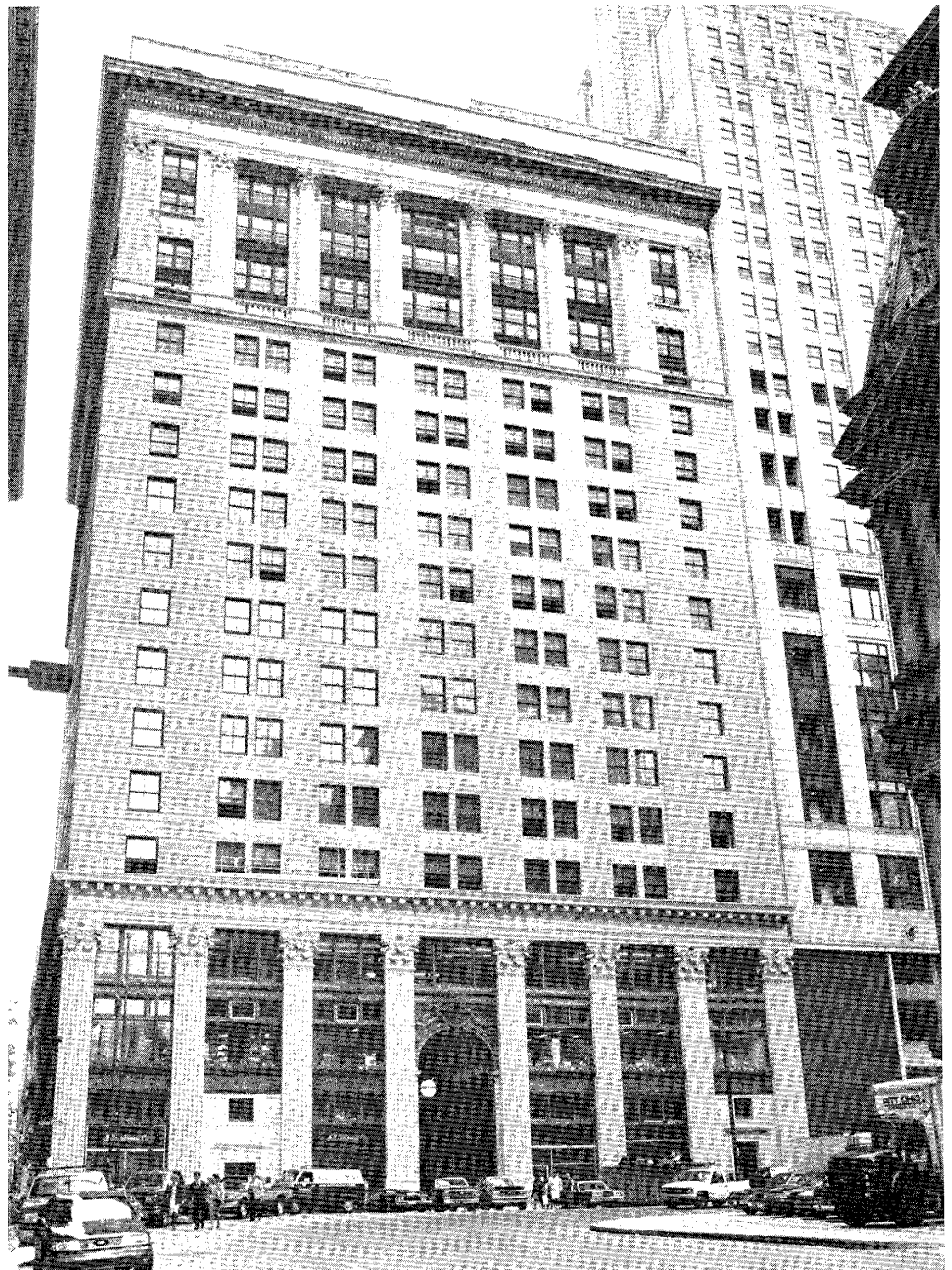
Figure 7. The South Penn Square elevation after its successful cleaning using the water soak method. Photo: Faherty/Kelter Associates, Inc.
