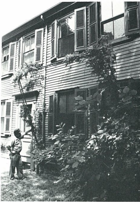
Figure 4. The pipe and strapping system, constructed with swivel sockets, allows the rigid support system to fold down away from the house. The strapping can also be removed from the pipe support for limited maintenance. Photo by Karen Day.
