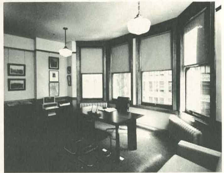
Figure 6. Typical 600 square foot office module after rehabilitation, with full ceiling height and one stand pipe radiator heat. Photo: Ron Gordon
