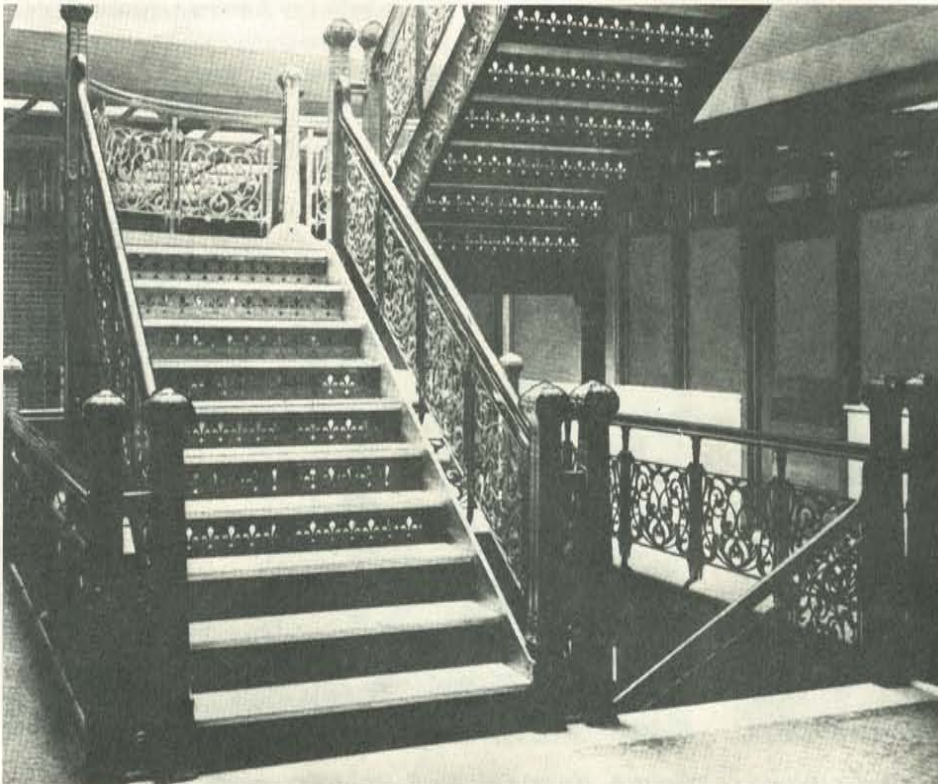
Figure 8. Burnham and Root's aluminum and bronze plated cast-iron stair remains the most notable architectural feature in the north half of the building. Minor repair work and a few missing elements have been replaced with cast aluminum. Favorable building codes allowed the open design.
