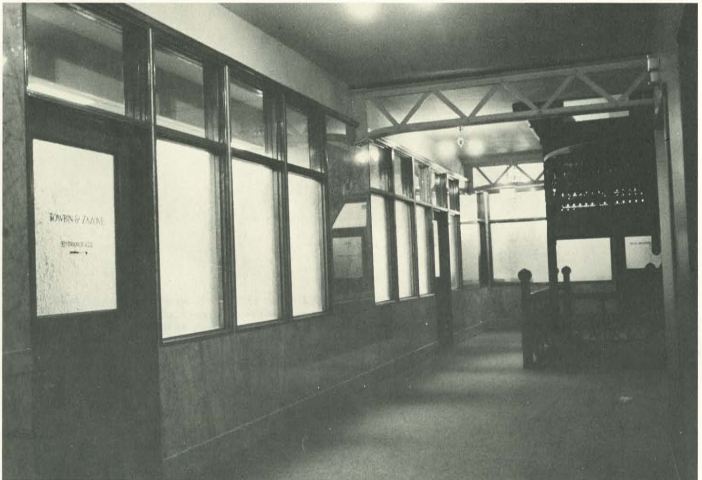
Figure 10. Rehabilitated corridor showing marble wainscot, oak and feather-chipped glass corridor partitions, full ceiling height and open ornamental stairs. Photo: Ron Gordon
