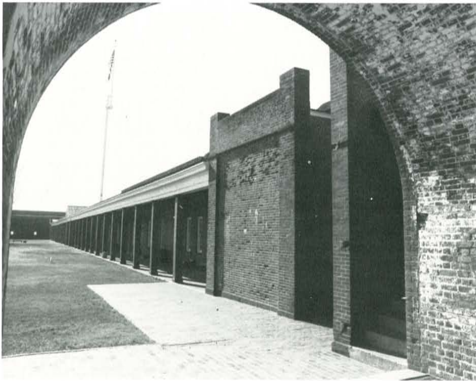
Figure 2. View from one of the open casemates, looking across a portion of the parade ground. The piazza provides a covered access to the enclosed casemates which flank the sally port. It was one of these enclosed casemates (each has a door and one or two windows) that was selected to house the museum object storage facility. Photo: Robert Darrigan
