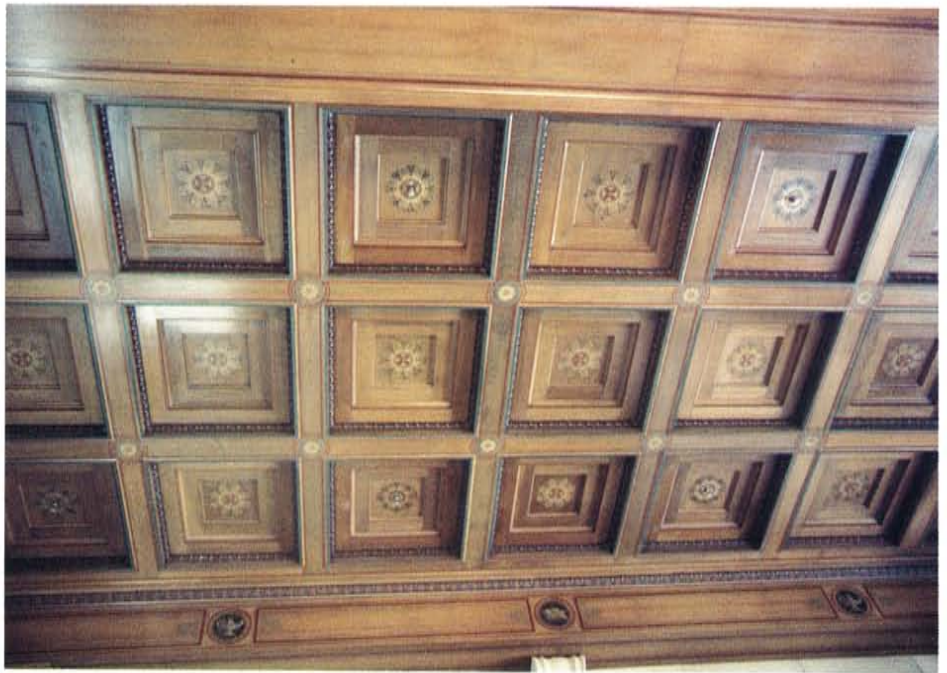
7. Following the work, the difference between the decal replacements and the historic stencilled panels is not discernible from the floor of the Central Search Room. Photo: Dell Corporation.
