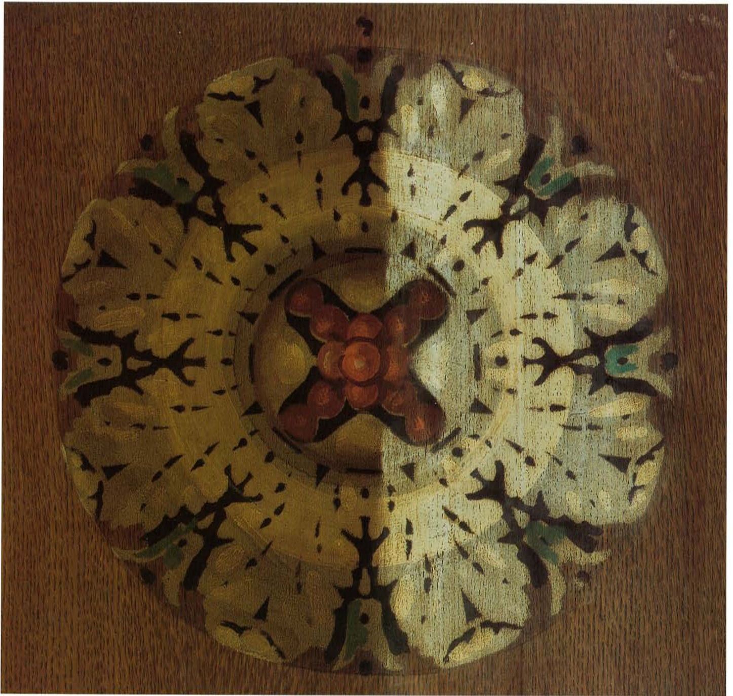
4. A historic stencilled panel was removed and cleaned in order to have a model for the replacement panels. In this view, only half of the panel has been cleaned, revealing the difference between the aged and original appearance of the ceiling. Since the ceiling was not scheduled to be cleaned, a decision was made to reproduce the original panel appearance and then artificially age the replacement panels to blend in with the existing ceiling. Photo: Dell Corporation.
