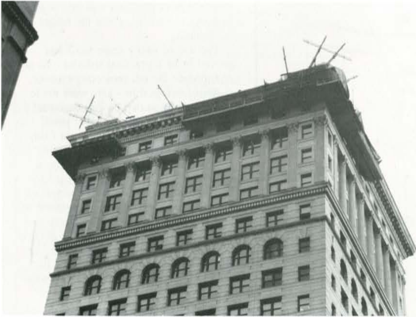
Figure 8. Access to the cornice was provided by cantilevered aerial scaffolds at the southeast and southwest corners of the cornice. All other locations were accessed by hanging two swing stages, side by side. The inner swing was hung off of a V-shaped bracket (shown) while the outer swing was hung from a steel deadman which projected horizontally across the cornice roof. Both the V-shaped bracket and the deadman were designed to transfer the weight of the swings vertically down through the center of the cornice. No load was placed on the outer edge of the cornice. Photos by Jeffrey S. Levine.
