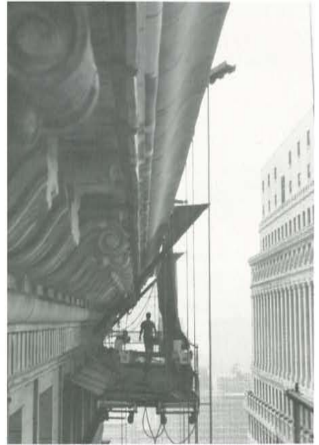
Figure 8. Access to the cornice was provided by cantilevered aerial scaffolds at the southeast and southwest corners of the cornice. All other locations were accessed by hanging two swing stages, side by side. The inner swing was hung off of a V-shaped bracket (shown) while the outer swing was hung from a steel deadman which projected horizontally across the cornice roof. Both the V-shaped bracket and the deadman were designed to transfer the weight of the swings vertically down through the center of the cornice. No load was placed on the outer edge of the cornice. Photos by Jeffrey S. Levine.
