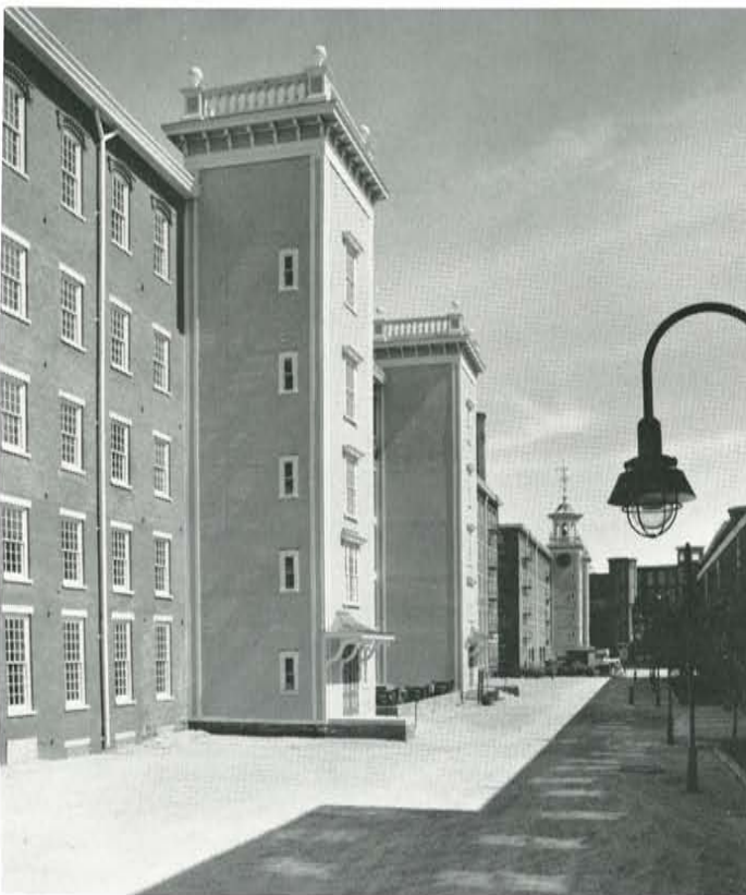
Figure 9. The window solution represents an important advance in the way in which aluminum windows can be designed to capture more fully the appearance of historic windows in larger buildings. Right photo shows wood sash in bottom row and aluminum in the upper three rows. Photos: Jim Higgins ©
