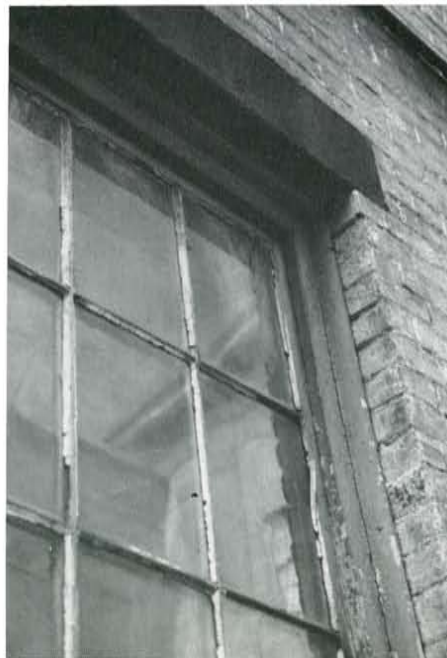
Figure 4. The decision to use an integral muntin for the outer glazing and a piggy-back interior glazing panel was an important component of the successful window solution. Sash shown before and after rehabilitation. Photos: Charles Parrott
