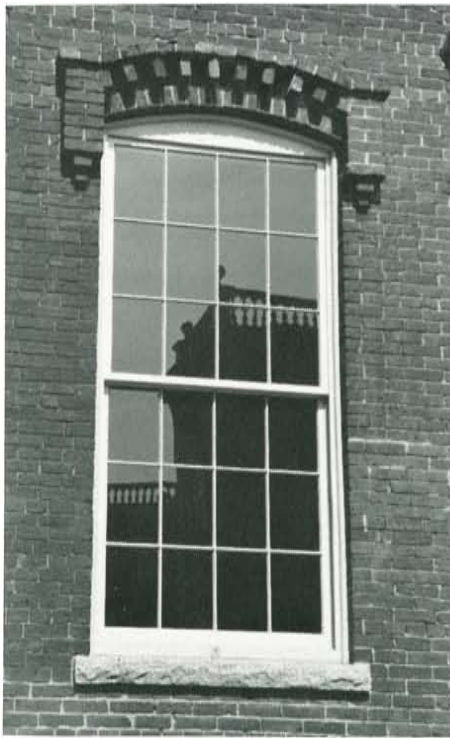
Figure 8. Replacement window sash after installation. Photo: Charles Parrott
