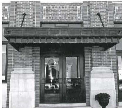
Figure 7. The new copper canopy on the east elevation of the Aldridge.
