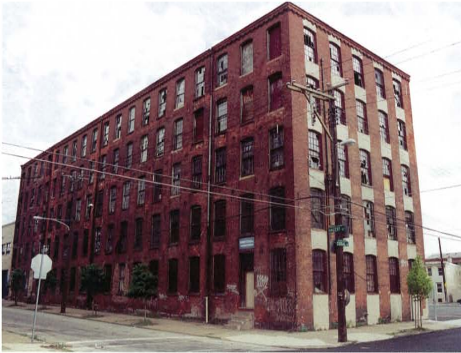
Figure 1. Constructed in 1886, the Beatty's Mill is located at a street intersection. The segmental arched windows are a distinguishing feature of the building.
