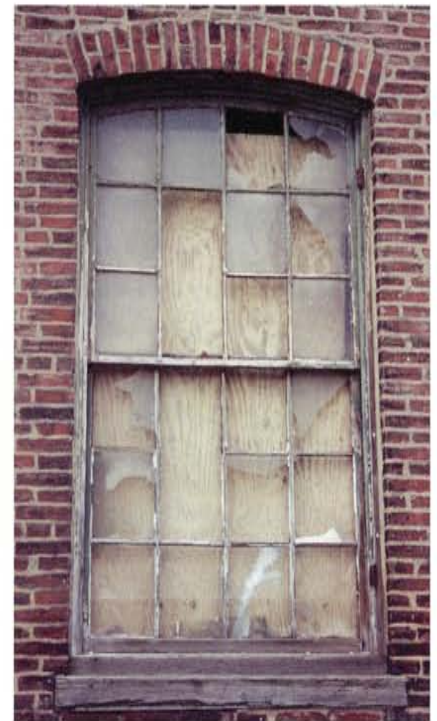
Figure 2. The historic double-hung wood windows had narrow sash and frame members that contributed to the distinctive qualities of the windows.
