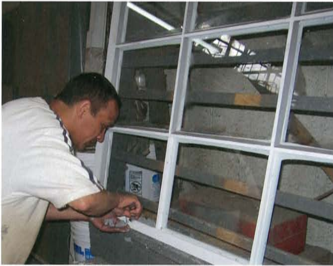
Figure 6. The outer glass was installed in the traditional manner, using exterior glazing putty. Photo: Charles Fisher.
