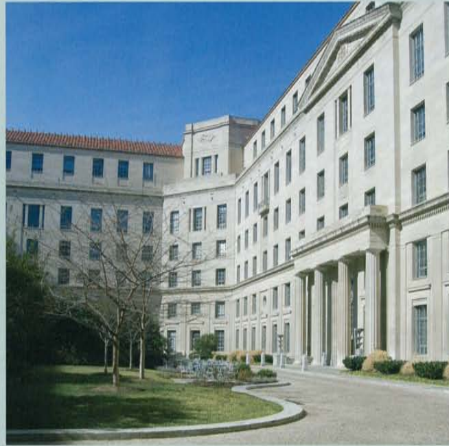
Figure a. In the primary courtyard within the U.S. Department of Justice Building, the aluminum windows emulate the appearance of steel windows with true divided lights. Depending on the floor level and location, the windows differ in size and consist of a varying combination of fixed lights, casements, and a hopper-style unit.
