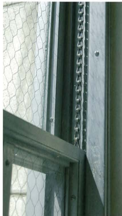
Figure 4. Early aluminum windows often mimicked wood windows in appearance and operations, even utilizing such details as parting beads, sash chains, and weights and pulleys. Photo of Folger Shakespeare Library in Washington, DC built in 1935.
