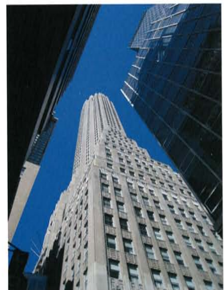
Figure 2. Aluminum windows gained early attention in part due to their use in signature buildings and to their appeal to Art Deco designers. Still one of New York's finest Art Deco skyscrapers, the original Cities Services Building projected a strong corporate image and utilized aluminum in many features, including the windows. (Photo: Shannon Koy.)
