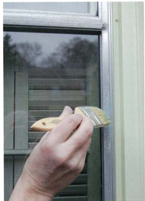
Figure 12. Cleaning tests may include a variety of products and methods such as mild soaps and detergents, etching cleaners, and abrasives. The gentlest means possible should be used, understanding that the goal is not to create a like-new appearance but rather to remove excessive grime and surface pollutants. Use of heavy etching cleaners or heavy-duty abrasives should be avoided on certain historic finishes. In this photograph a mild etching cleaner in jell form is being tested on a storm window with a mill finish.
