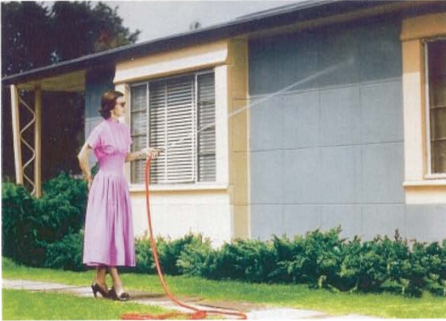
Figure 11. Aluminum windows were described as a perfect choice for Lustron Homes because of their modern appearance and ease of maintenance. Along with the procelain-enameled-steel exterior wall panels, the manufacturer claimed that the only cleaning and maintenance materials required for a Lustron Home were "soap, water, and a damp cloth." Today, cleaning is recommended for any historic aluminum window as part of a cyclical maintenance program.
