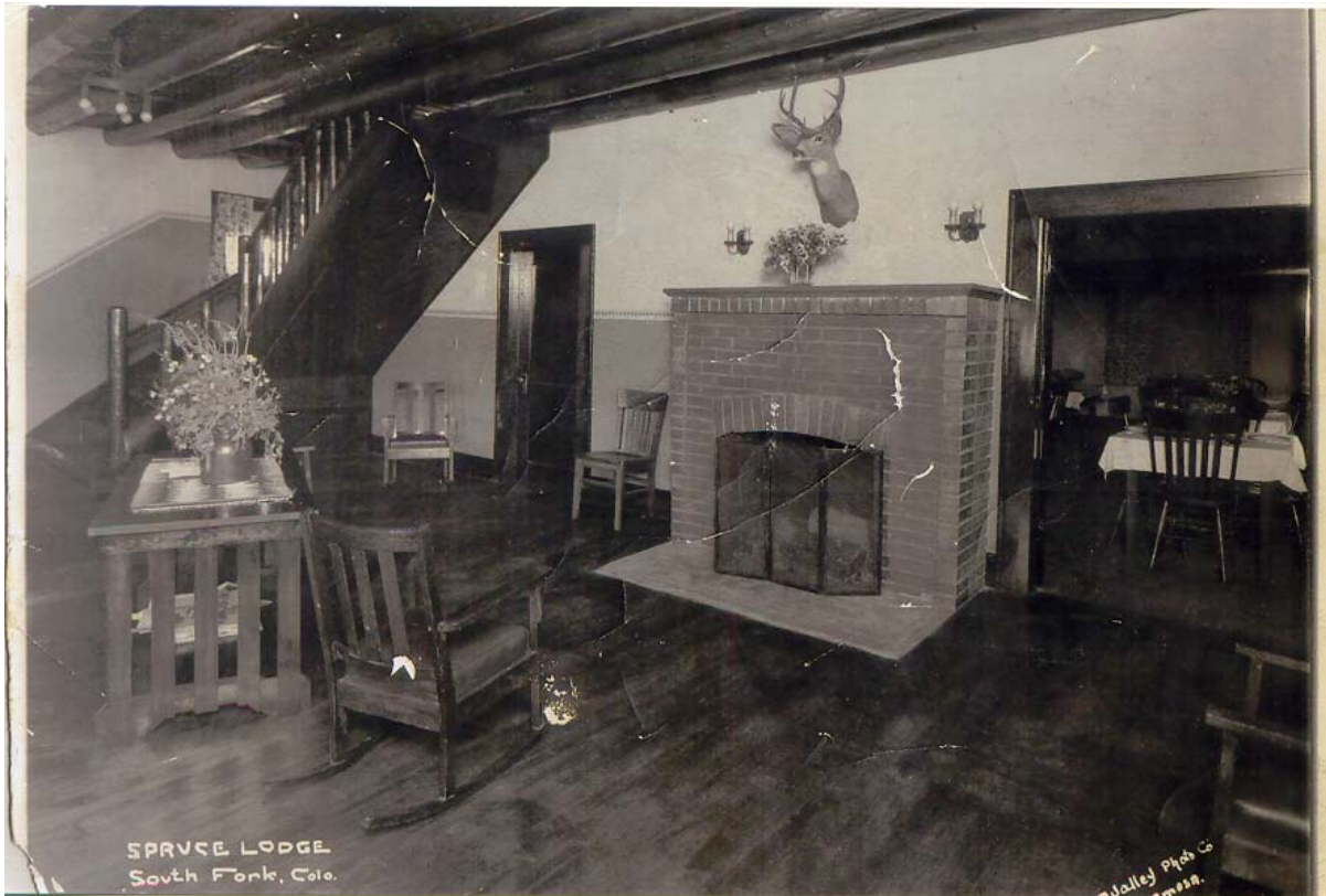
Photo No. H3: This 1938 photograph shows the lodge's lobby and the appearance of the fireplace before being covered with stone.
