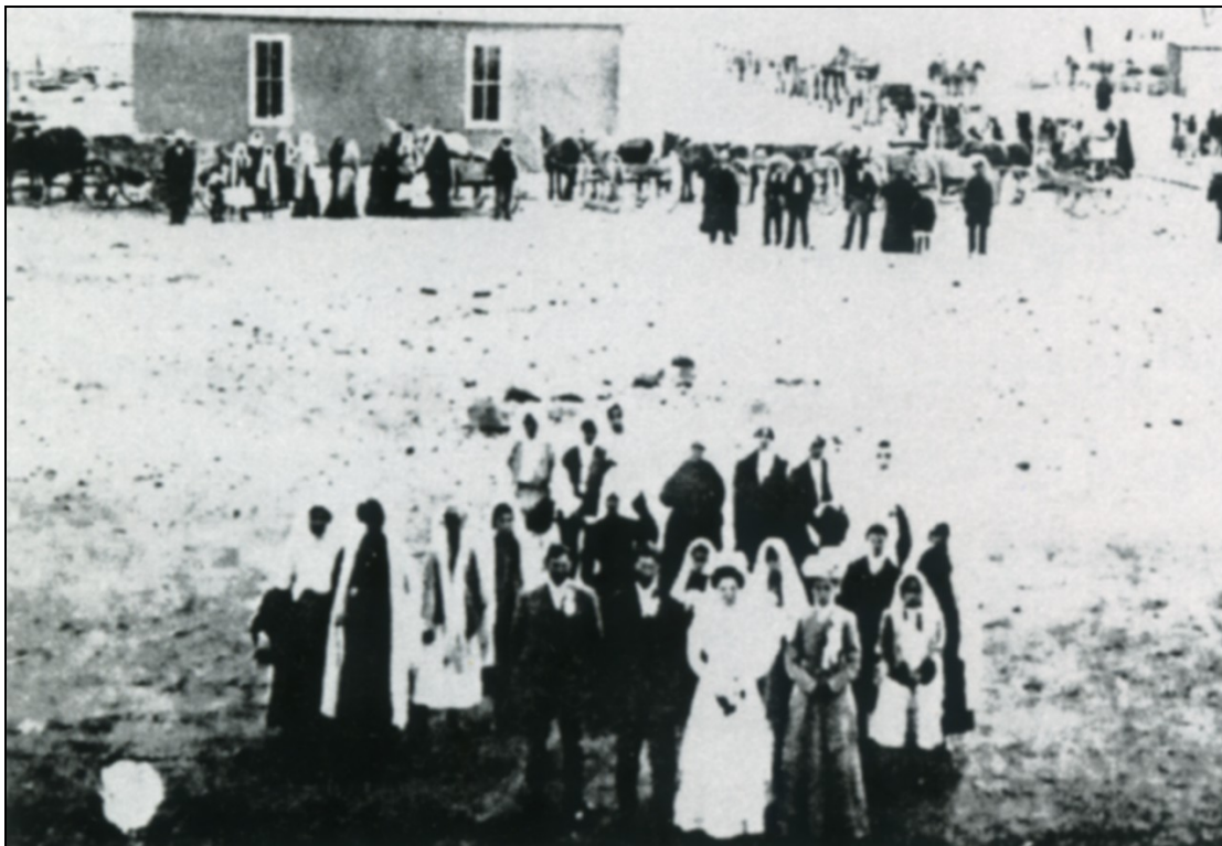
Figure 2. This ca. 1912 photograph of a wedding party shows the 1878 adobe church at Capulin in the background with the current church under construction at the upper right. Courtesy of 100 Year, 1912-2012 Anniversary Jubilee (2012), 2.
