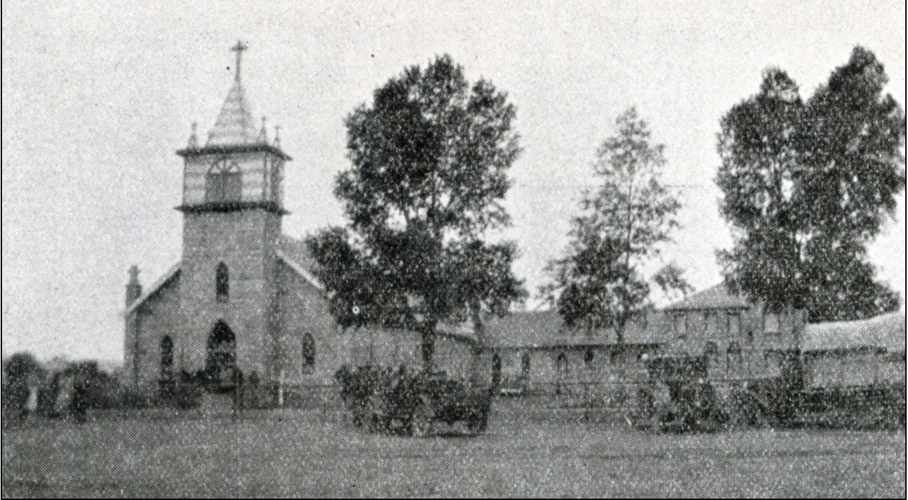
Figure 5. By 1934 the church displayed its current tower (1928), as well as north additions: the one-story stone chapel (ca. 1913-17) and the ornamental concrete block chapel expansion (one-story) and rectory (two-story) (both 1933-34). The view in the photograph is to the west-southwest. Courtesy of El Reino de Dios a La Parroquia de Conejos en Sus Bodas de Diamante (1934), 22.
