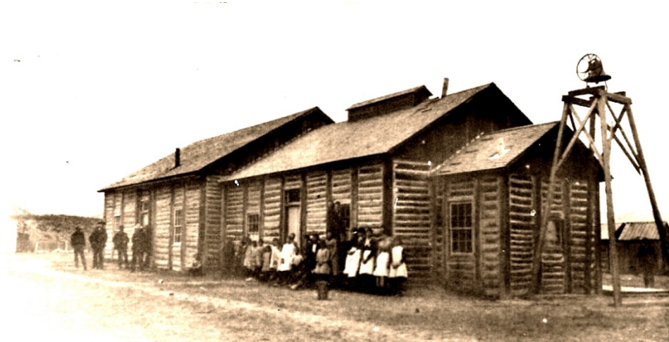
Figure 1: Log building erected in 1880 by the U. S. Army and used as a hospital as part of the Camp on White River. The building was later used as a school, as Rio Blanco County's first courthouse, and for other community purposes, circa 1890, courtesy of Rio Blanco County Historical Society and White River Museum.
