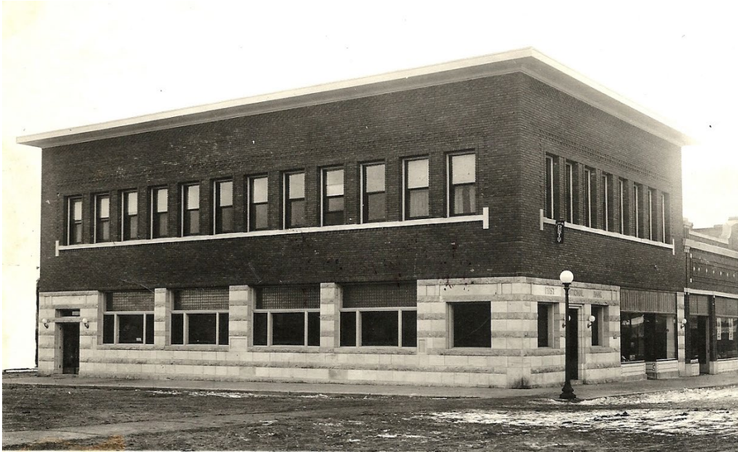
Figure 15: First National Bank Building, 504 Main Street (5RB.2238), view to southwest, circa 1920, courtesy of Rio Blanco County Historical Society and White River Museum.
